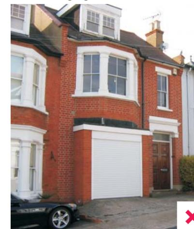
The installation of this garage has resulted in the negative loss of the ground floor bay ✗
